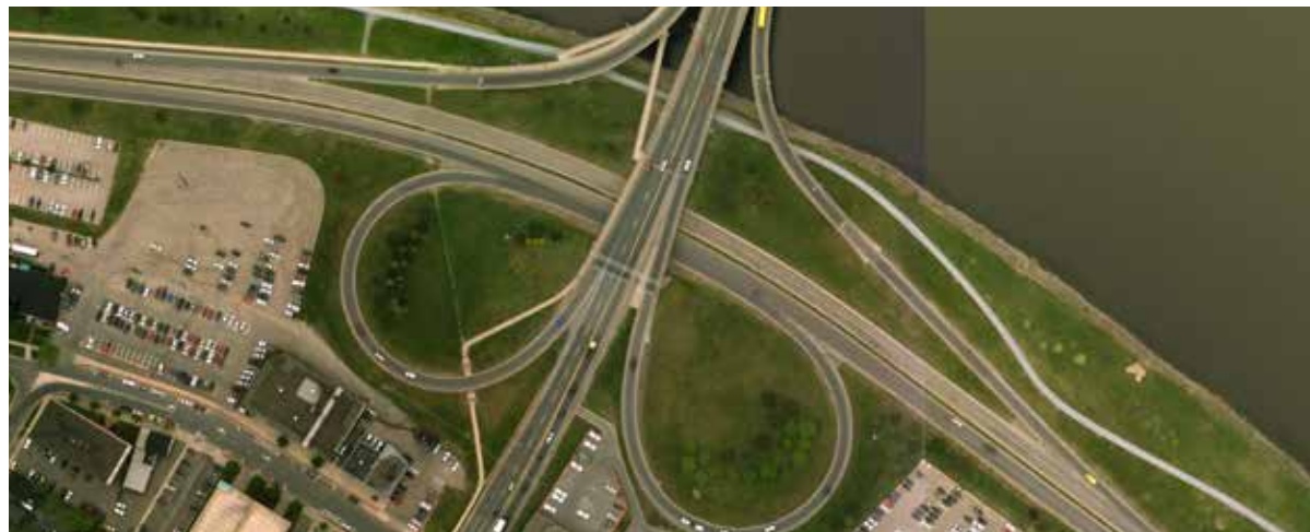
Westmorland Street Bridge and on-ramps
