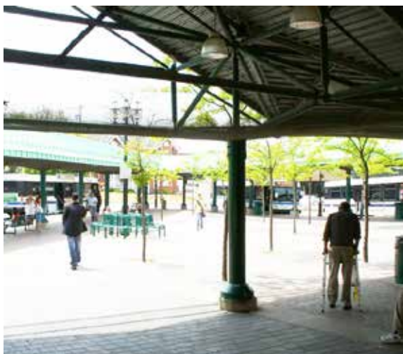
Integrated transit facility in Barrie, Ontario
