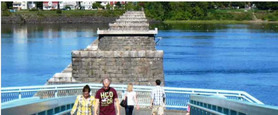
The Carleton Street Bridge piers
