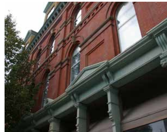
Architectural character of Queen Street
