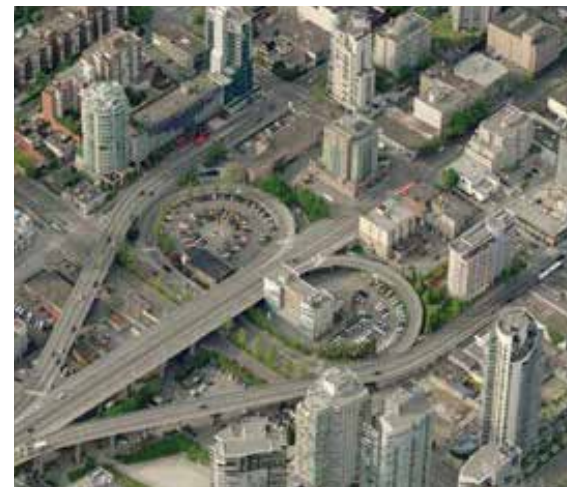
Existing Granville Street Bridge
