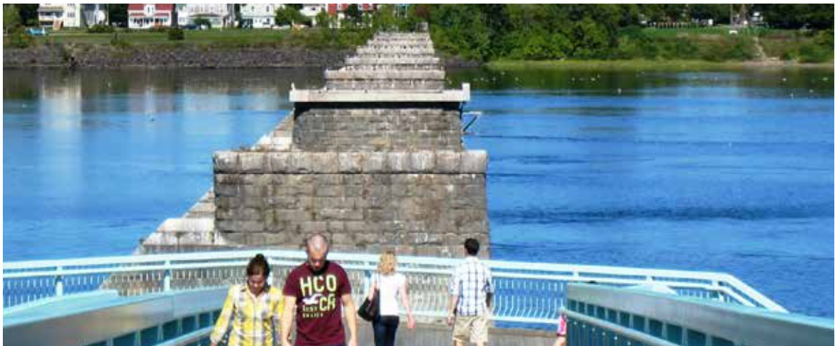
The Carleton Street Bridge piers
