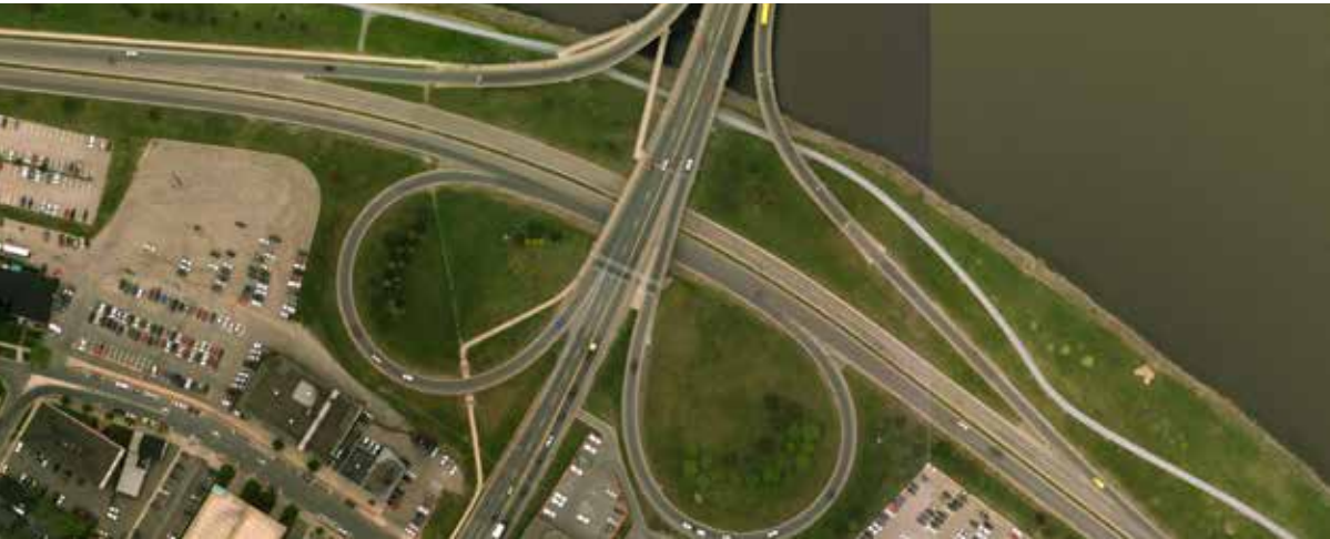
Westmorland Street Bridge and on-ramps
