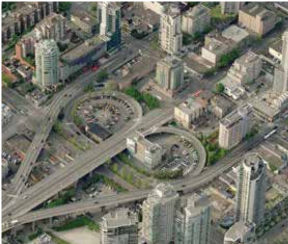
Existing Granville Street Bridge
