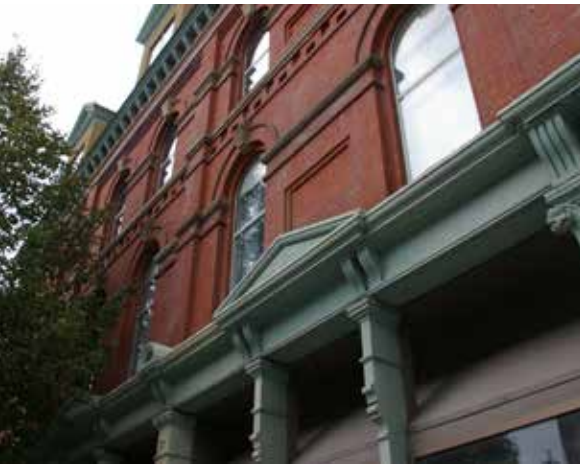
Architectural character of Queen Street
