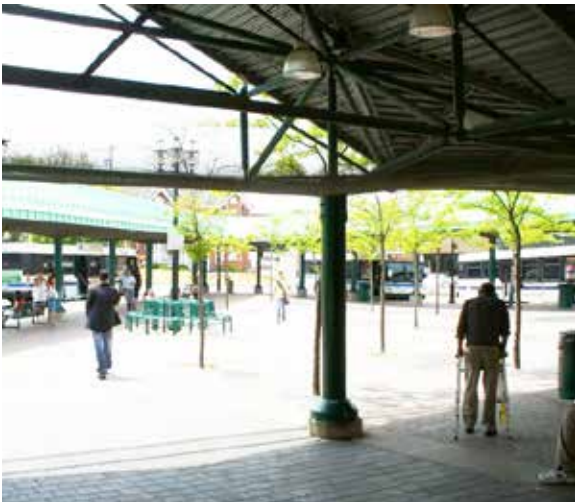
Integrated transit facility in Barrie, Ontario
