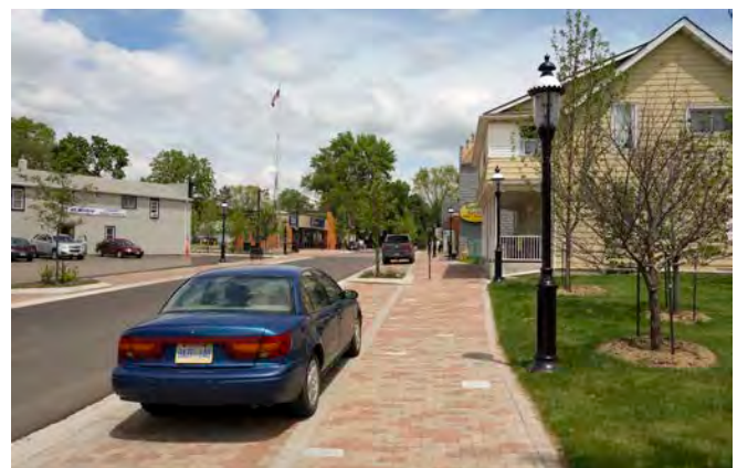
Examples of on-street parallel parking with a unit paved surface at sidewalk level, with a mountable curb.
