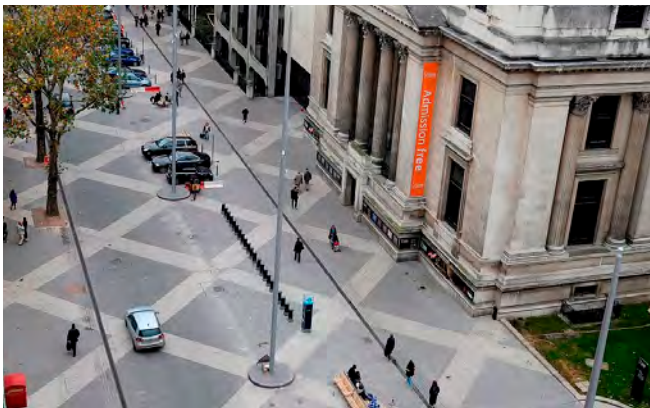
2. Unit paved sidewalk with rolled curb and unit paved road for Shared Streets
