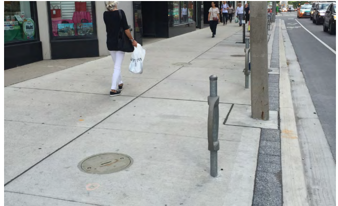
4. Concrete sidewalk with narrow unit paver band for Downtown Commercial Streets
