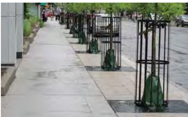
3. Concrete sidewalk with wide unit paver band for High Streets
