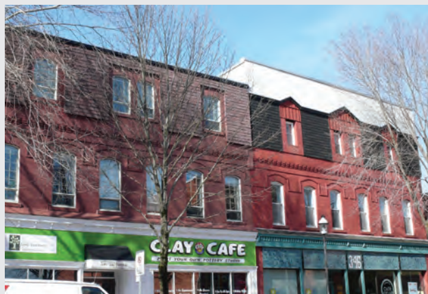
Inexpensive materials (including roof shingles) used as cladding in these contemporary retrofits creates a stark contrast with the original masonry and detailing.
