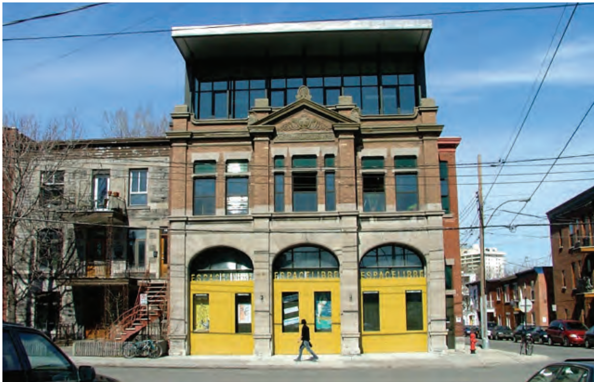
This contemporary rooftop addition is stepped back from the heritage facade, and designed with vertical proportions.
