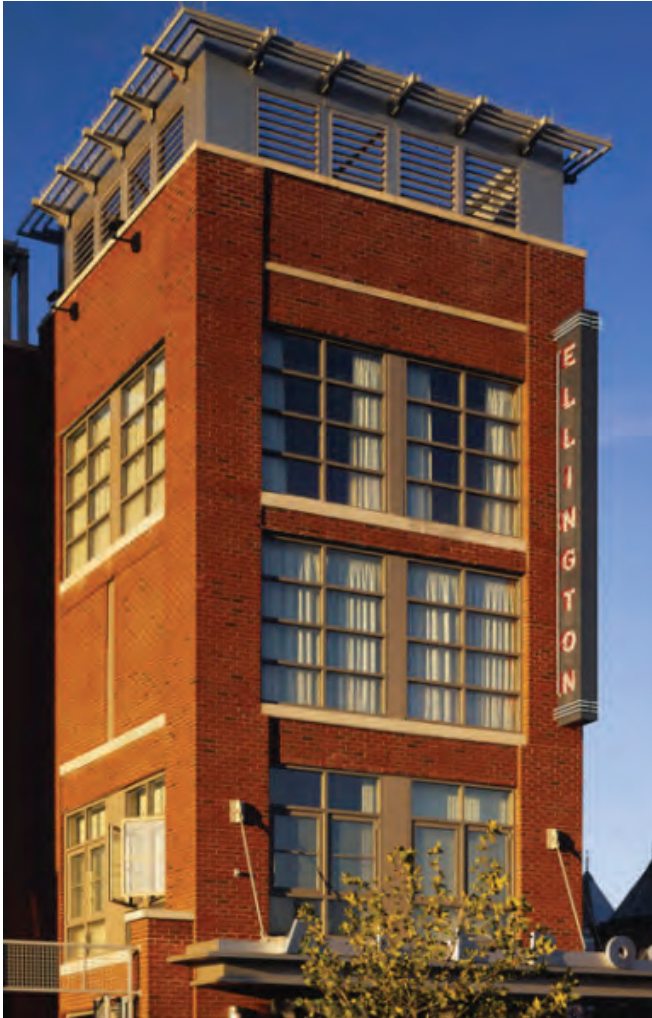
Roofline treatment creates a strong building top, a memorable architectural treatment, and screens rooftop mechanical equipment.
