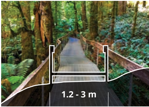
Raised Boardwalk, Guided Wire Mesh/Wood Surface
