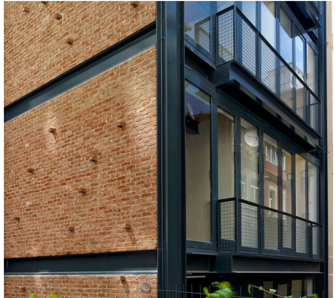
Steel structural system expressed through facade design.
