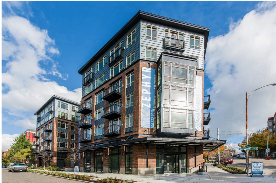
Mixed Use Apartment Project, Seattle
