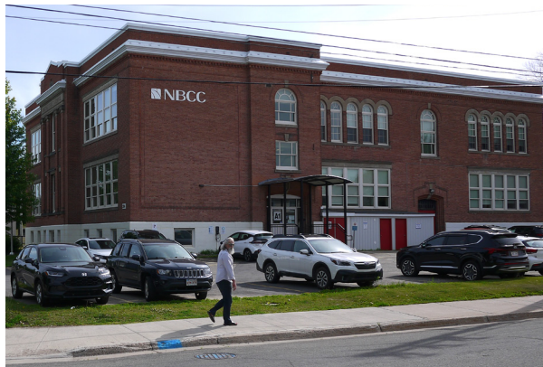
Former Smythe Street School adaptively reused and converted into corporate offices
