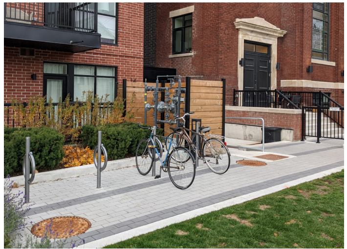
Screen and planting around gas metres
