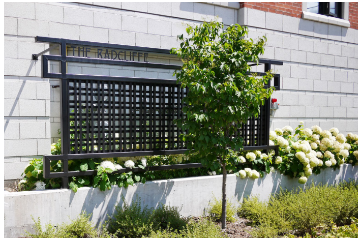
Screening of utility meters next to a building entrance
