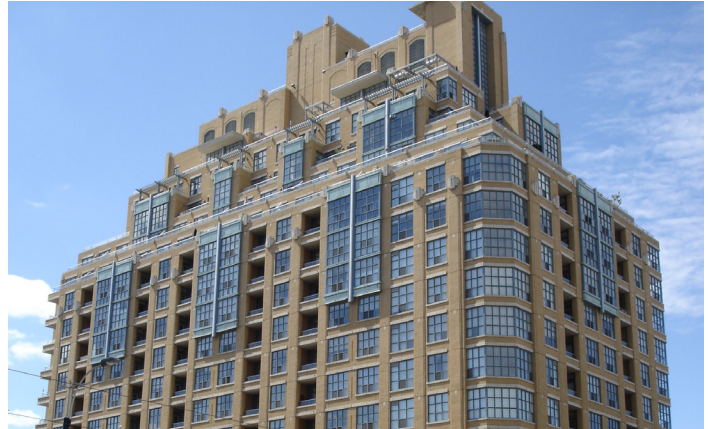
Interesting rooflines and rooftop mechanical integrated into design
