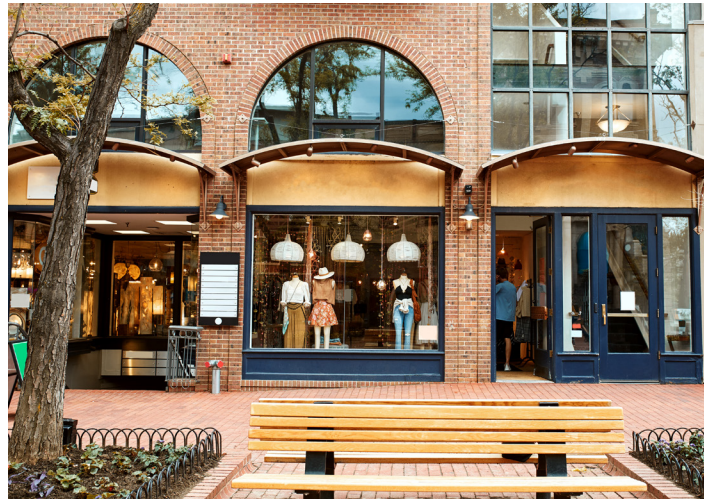
Articulation of a façade with vertical rhythm of bays, windows, and canopies
