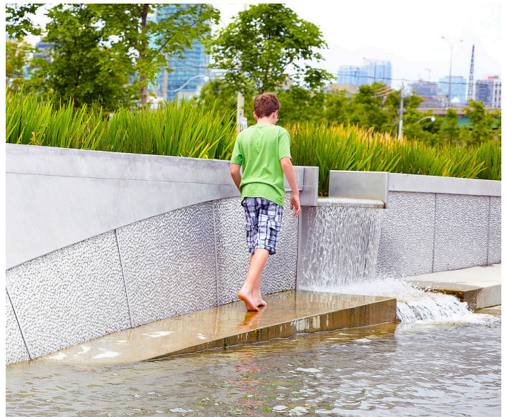
Example of an innovative stormwater management facility.
