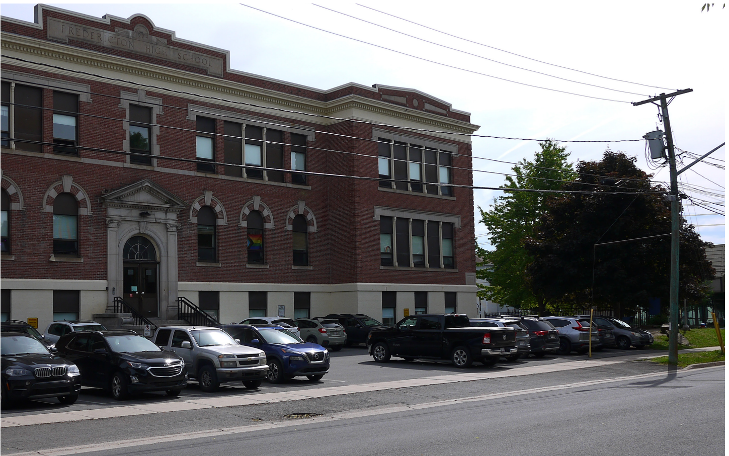
Primary gateway at George Street Middle School
