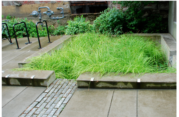
Curb cut allowing rainwater runoff into planting area, Portland, OR
