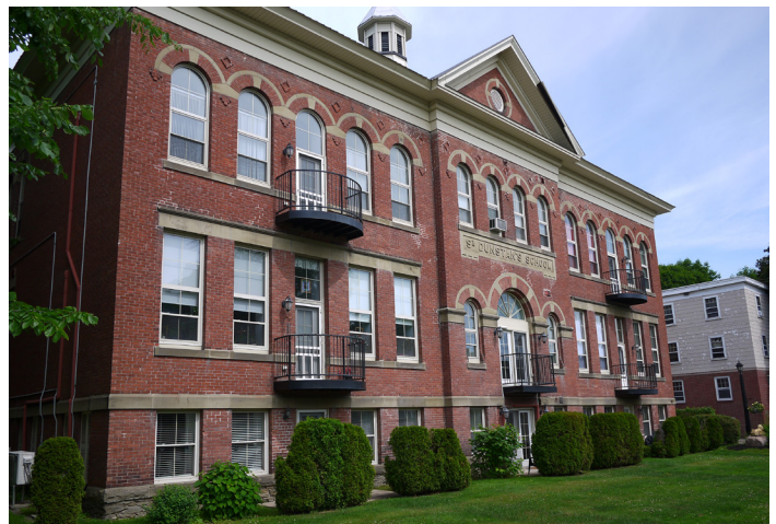
Former St. Dunstan's School on Regent Street adaptively reused and converted into apartments
