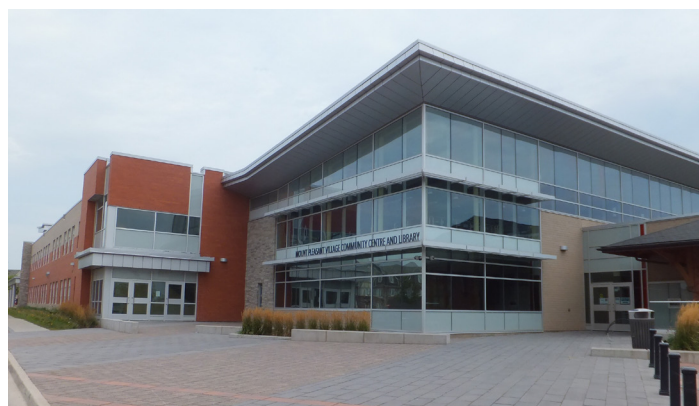
Example of the use of architectural features to denote landmark community facilities
