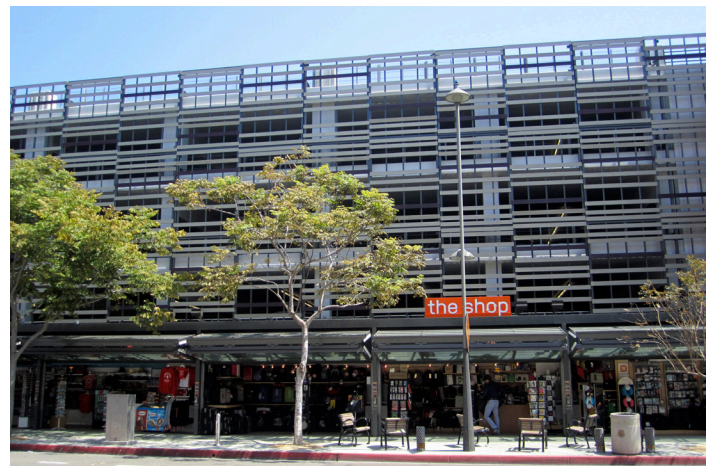
Parking structure with rhythmic façade design (image: La Citta Vita, CC BY-SA 2.0, Flickr)
