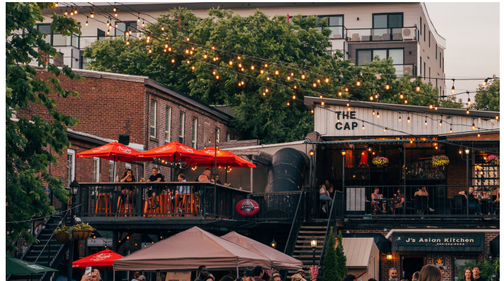
Signage integrate into a sign band as part of the façade design
