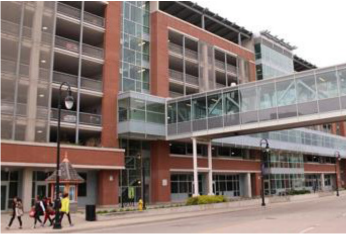
Parking structure with retail uses facing street at ground level
