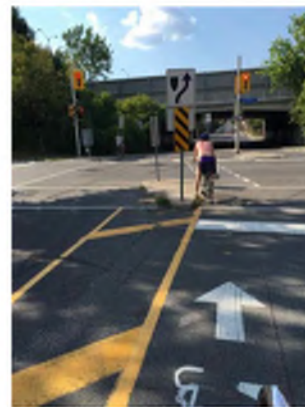
Photo showing "chicken tracks" through intersection
