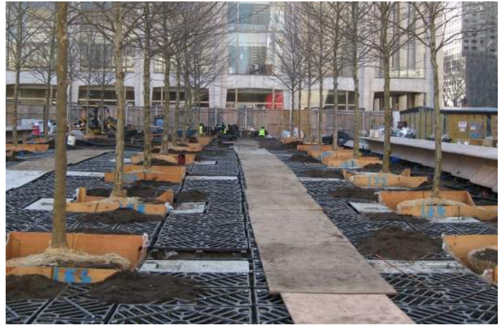
Soil cell installation at Lincoln Center New York (Source: DeepRoot on Flickr.com)
