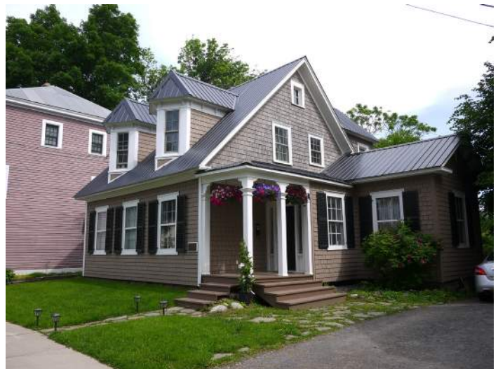
Use of dormers and gables
