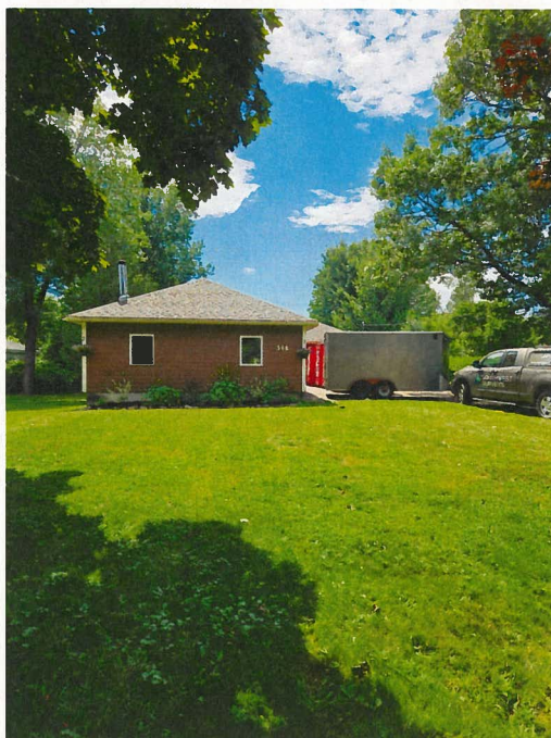
Front - Gibson Street (West) / Façade – rue Gibson (ouest)
