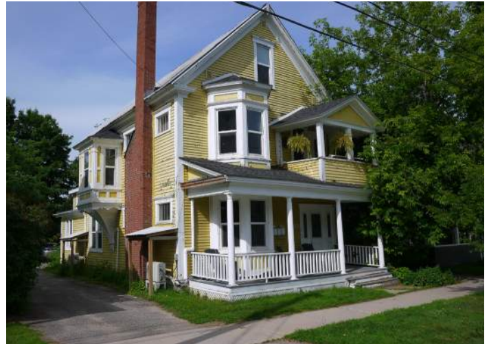
Typical building in the Neighbourhood Area
