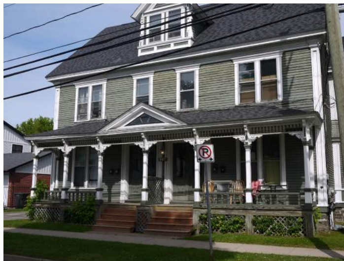
Porch feature for a multi-unit building
