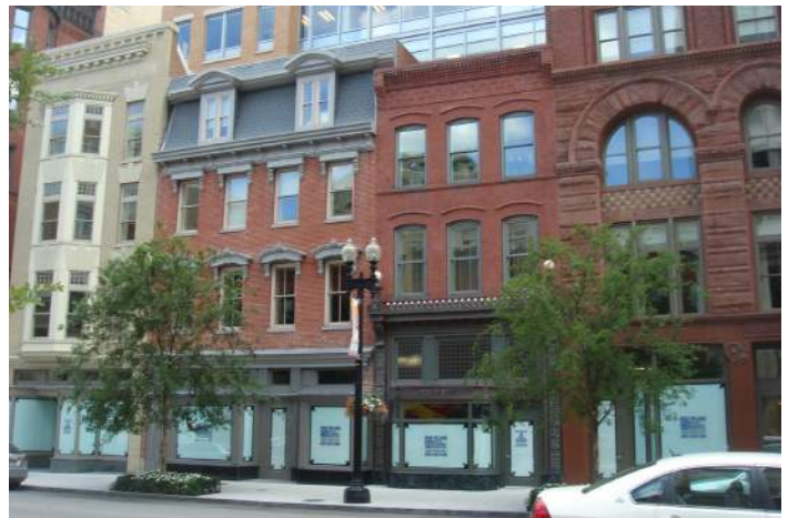
Preserved façades in a large redevelopment
