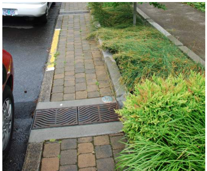
Bioretention planters for stormwater management, Portland OR
