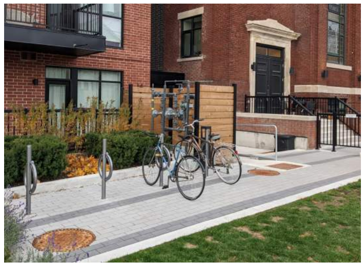
Screen and planting around gas metres
