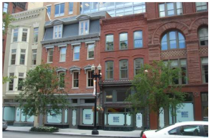
Preserved façades in a large redevelopment
