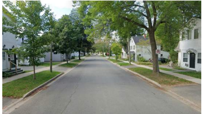
Existing conditions on Charlotte Street
