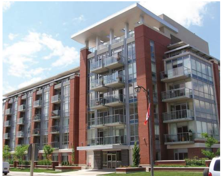
Architectural expression emphasizing main entrance location
