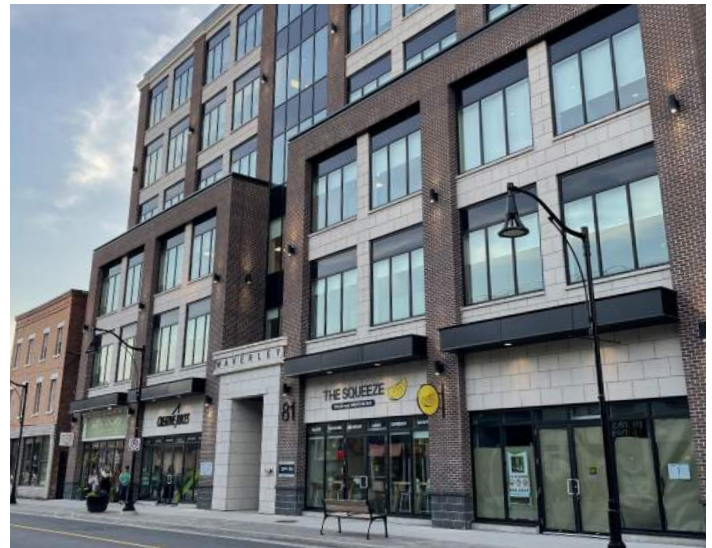
Mid-rise building with a 3-storey street wall
