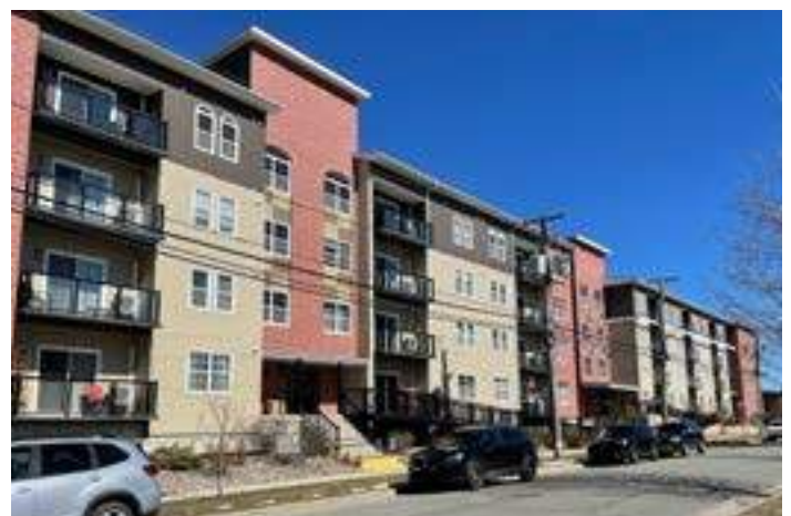
Redevelopment example in the Rail-Adjacent Character Area
