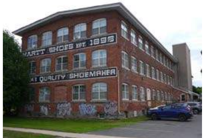
Heritage industrial building in the Rail-Adjacent Character Area
