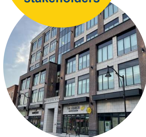
Mixed-use building in the South Core
