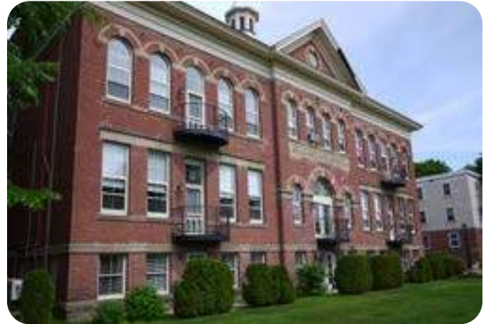
The former St. Dustan's Elementary School re-purposed for residential units.
