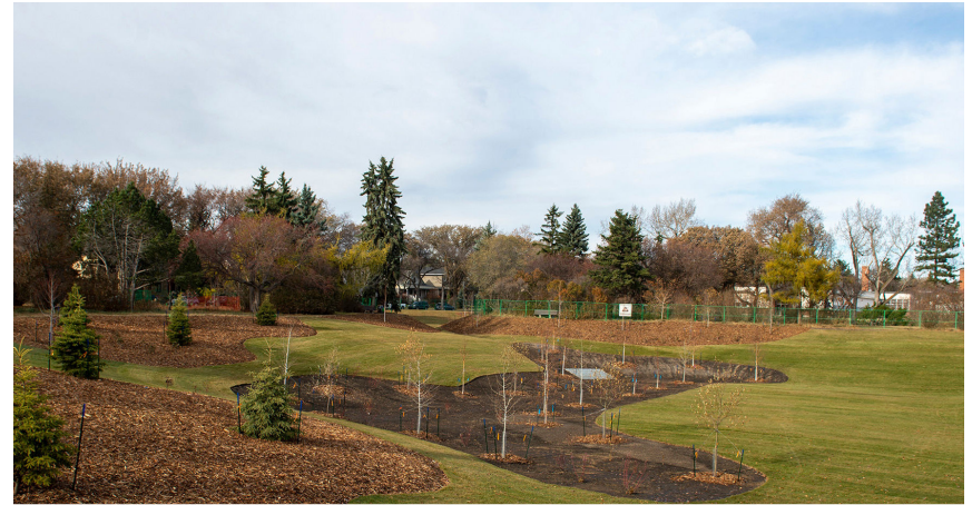
Figure 15: A park space is designed to function as a dry attenuation pond in Edmonton, AB (Image source: EPCOR)
